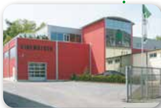
high-bay warehouse & administration
